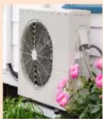
Air Source Heat Pumps
